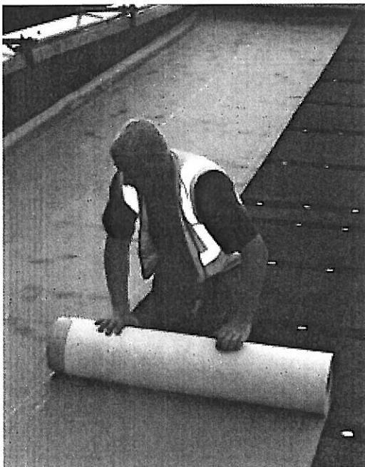
Materials supplied by Proos Roofing Supplies, Birmingham.
